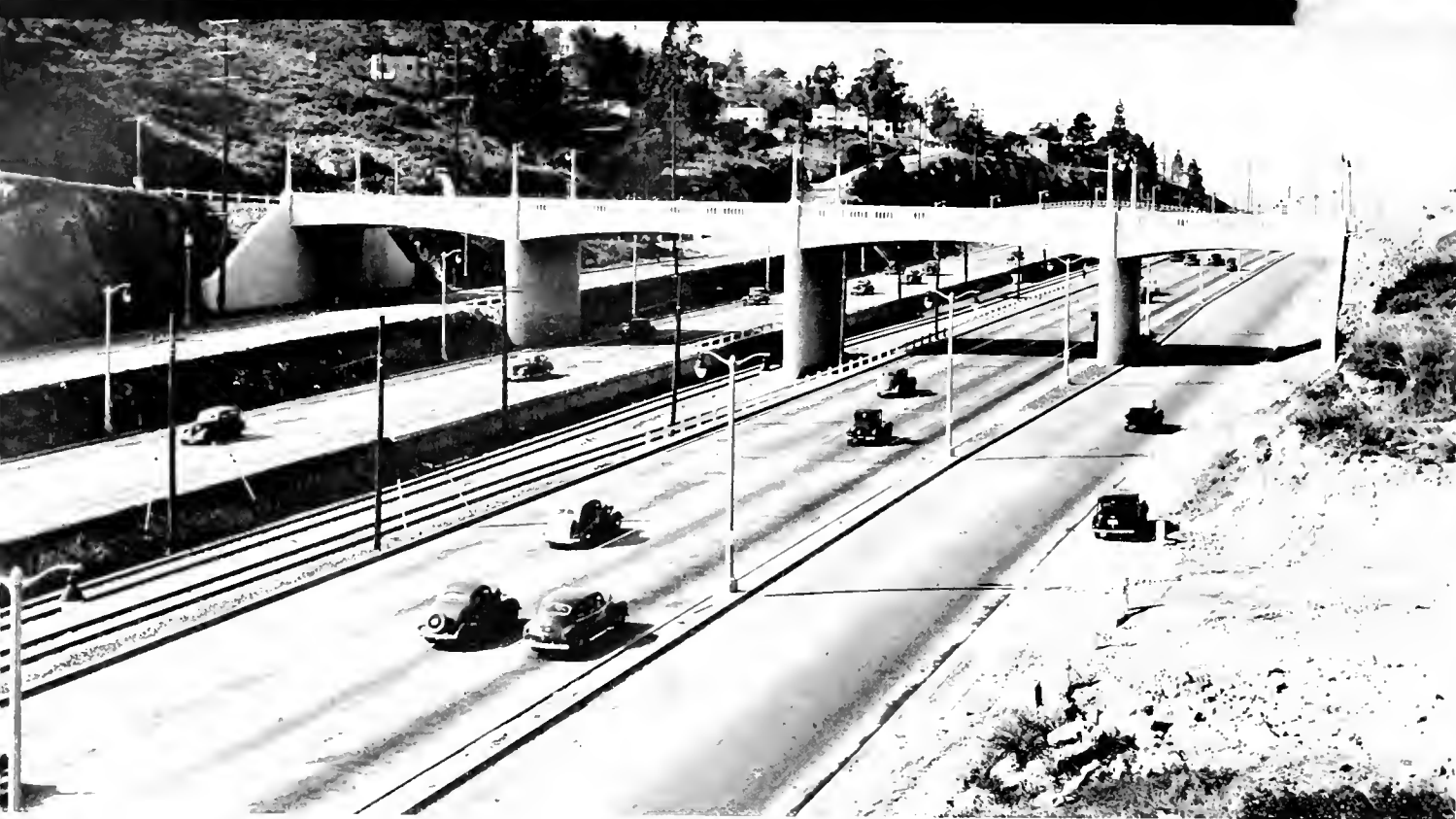
Completed section of U. S. 101, a six-lane freeway through Cahuenga Pass with which proposed Hollywood Parkway will connect
